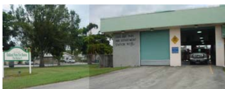
Station #09: 301 NE 38th Street
