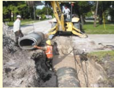
Installing new drainage pipes on NE 34 Court for NE 5 Avenue Project
