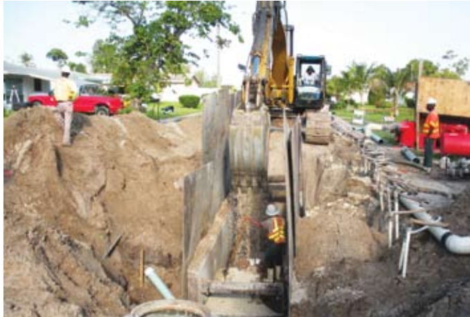
Sewer main installation along NW 27 Street.
